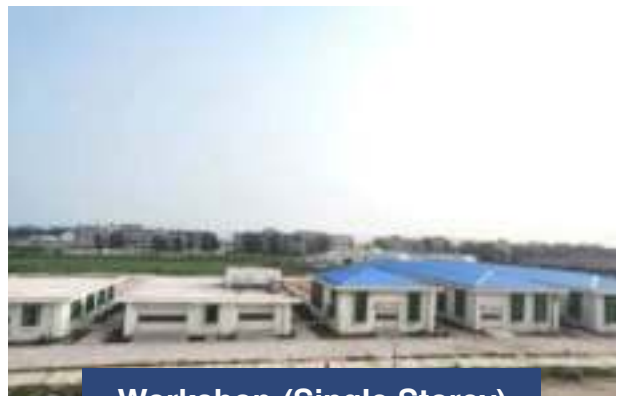
Workshop (Single Storey)
