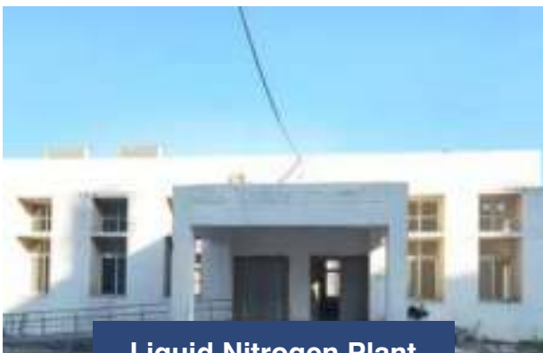
Liquid Nitrogen Plant
